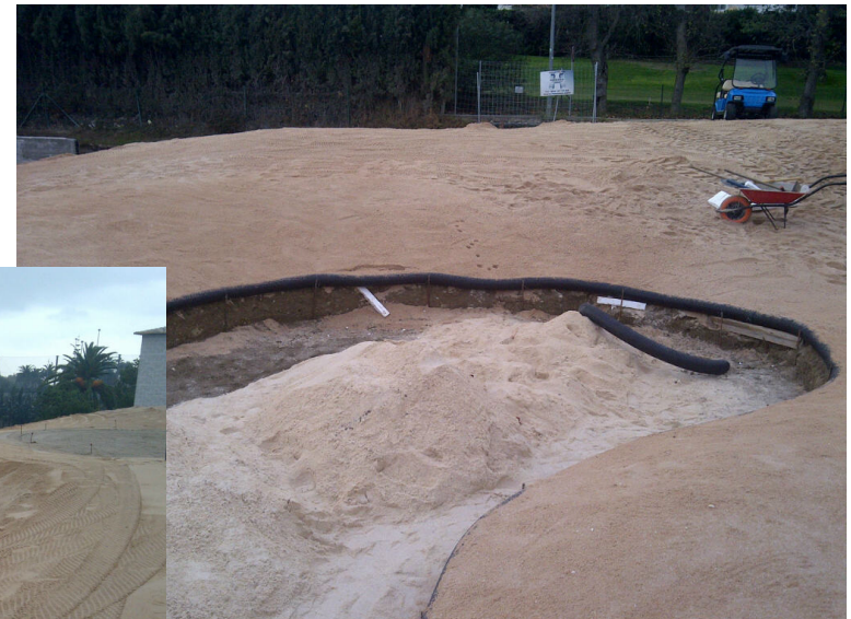
Bunker construction and soil around the green
